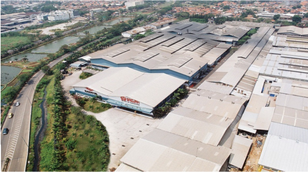
Kapuk Plant (Radiator Facilities)
